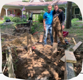
rebuilt walkway & stairs
