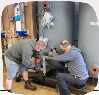
well hook up complete
